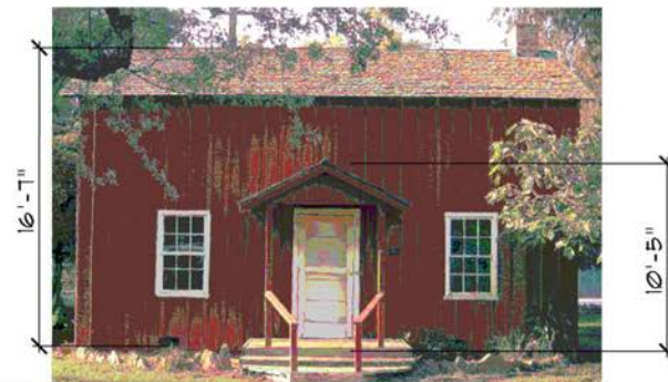
CRAMER HOUSE FRONT ELEVATION SCALE: 3/8"=1'-0"
